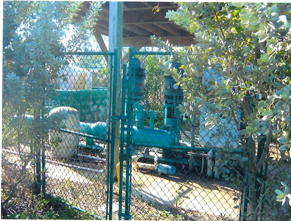
View of Pumphouse
