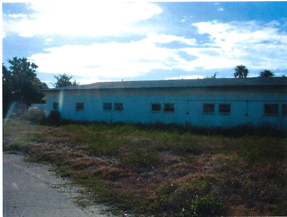
Existing Maintenance Building Looking Southeasterly
